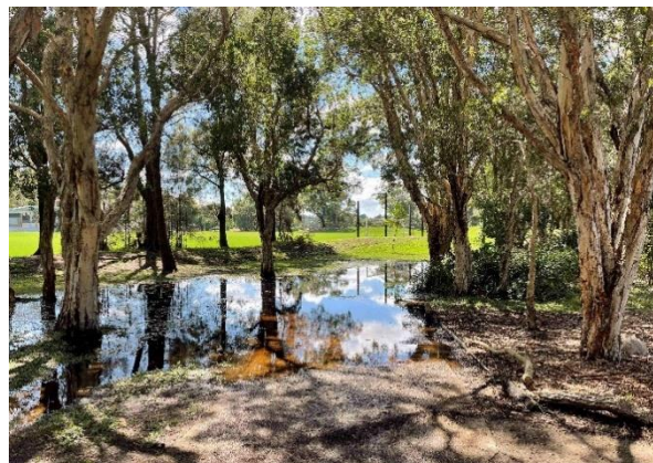
The shared path at Ewen Park floods regularly – a raised path is a possible solution
